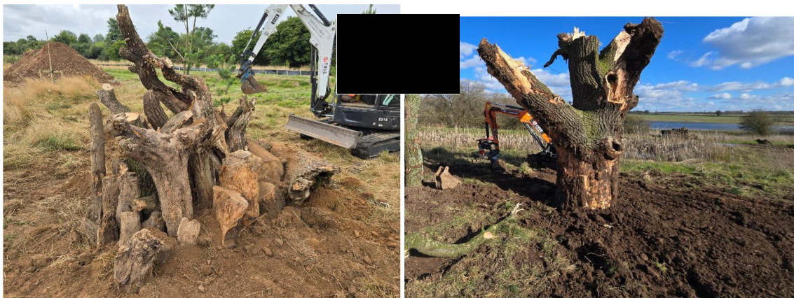
Image 22: Vertical log piles
